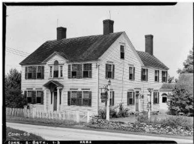
A multifamily housing example in Bethany
